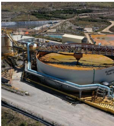
Water Treatment at Lagunas Norte Mine
