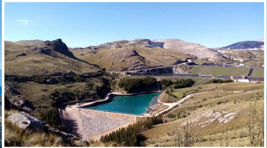
Lagunas Norte ARD Water Sedimentation Pond
