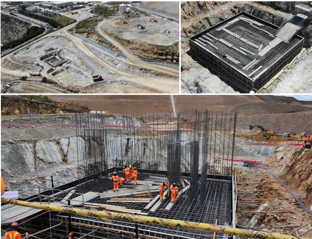
Figure 1. Ball mill and scrubber foundation works at Lagunas Norte mine
